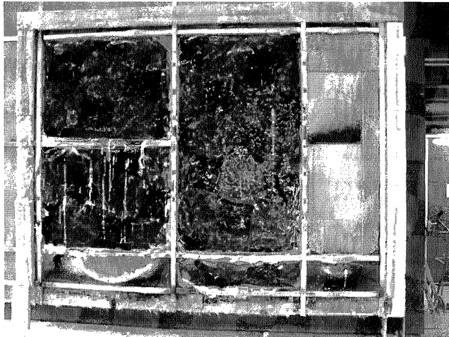
Photo 13: Fire side of curtain wall after the test.
