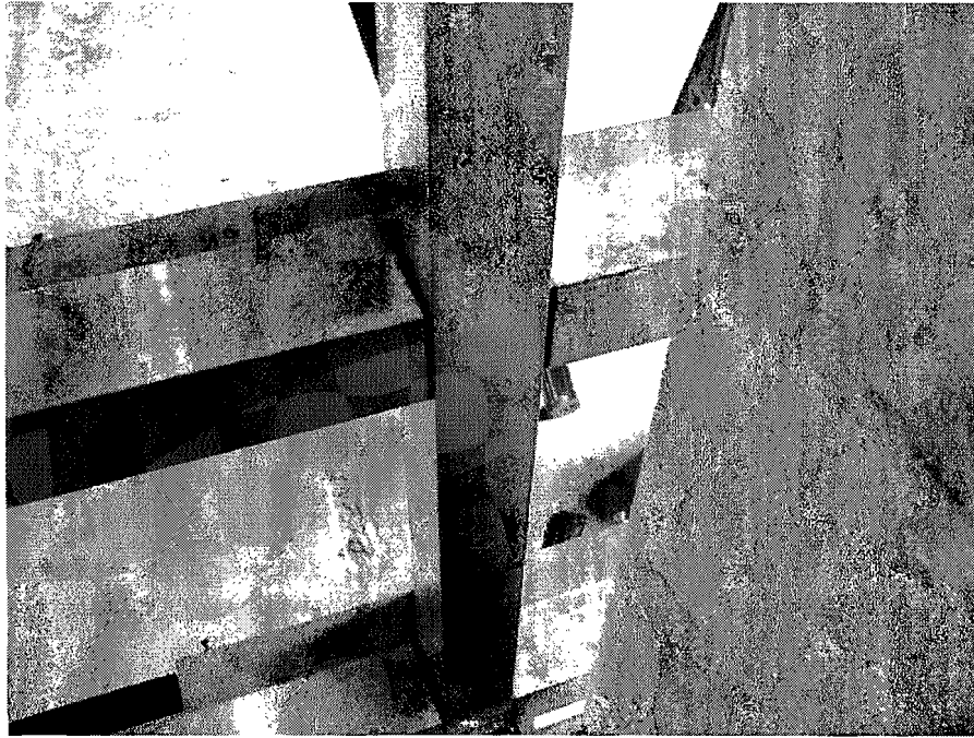
Photo 3: Junction of the structure.
