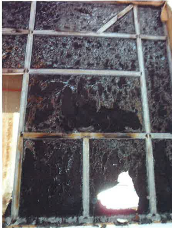
Photo E (bottom) Element after test and cool down on the exposed side.
